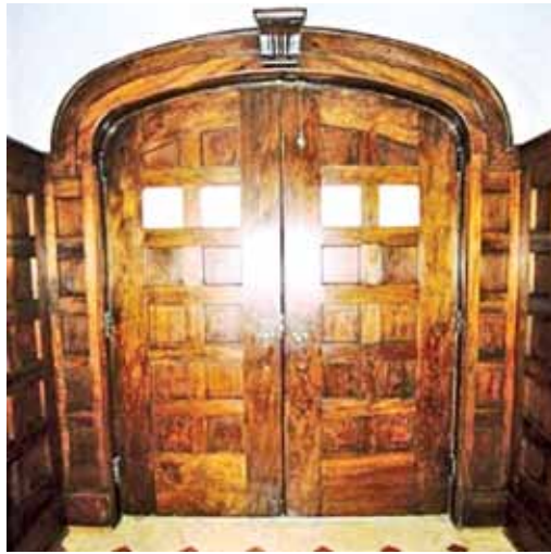
Front doorway is original design.
