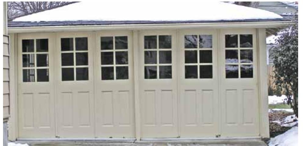
Old doors on garage are still intact.
