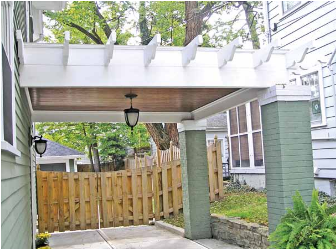
Pergola was completely rebuilt.
